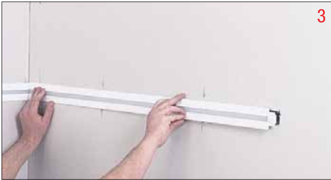
Cut Channel and Mount to Studs with Screws
