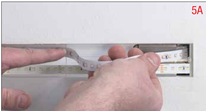
5A Add LED Strip Flat in Channel and Snap in Lens (Room Wrapping Installation, Pg. 36)
