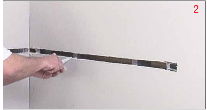
Cut Out 5/8" Thick Drywall
