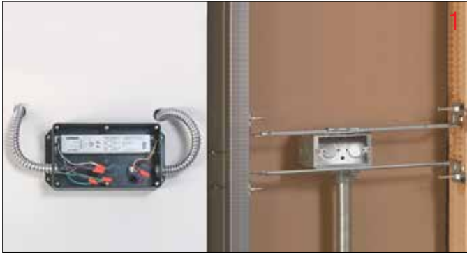
Install Remote Power Supply and TruLine .5A Junction Box
