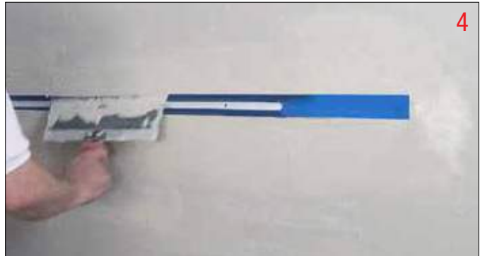
4 Plaster and Paint
