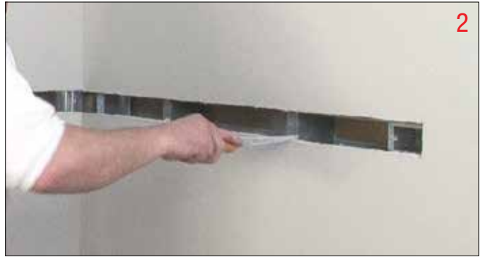
2 Cut Out 5/8" Thick Drywall
