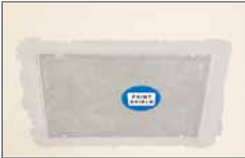
Contractor plasters fixture
