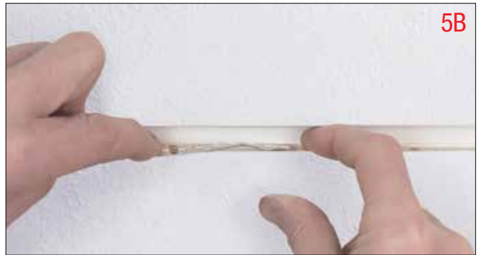
Add LED Strip on Side of Channel and Snap in Lens (Picture Frame Miter Installation, Pg. 20)
