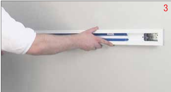
3 Cut Channel and Mount to Studs with Screws
