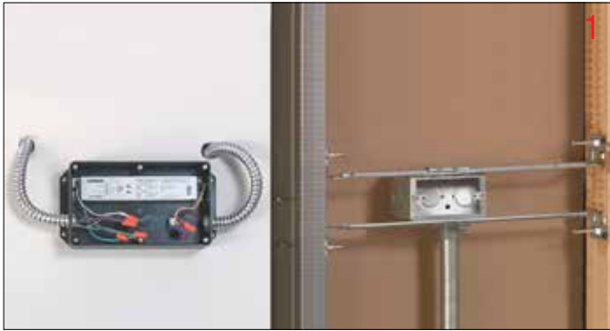
1 Install Remote Power Supply and TruLine 1.6A Junction Box
